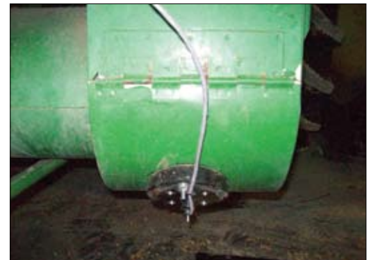
John Deere FG Installation
